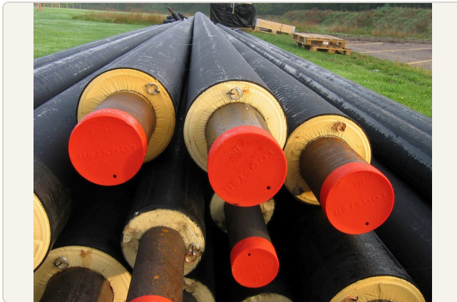
Mike1024, „Pre-installation insulated underground pipes for district heating”, Wikimedia Commons, public domain – resized · Anatomy of a pre-insulated pipe: water in the foam multiplies the heat emission.
